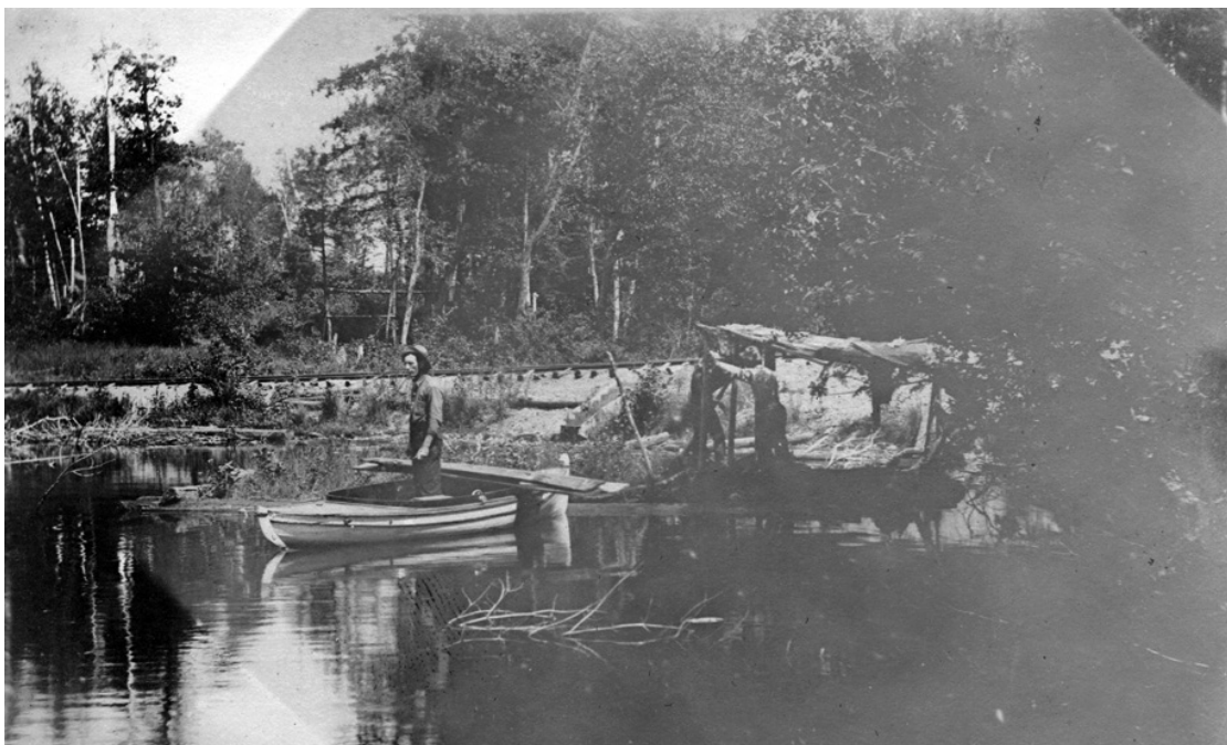
Figure 14. The only known photograph of the Brown Brothers logging railroad as it crosses the bog separating Black Oak and Dollar Lakes (August, 1908). After tearing out the rails in 1909, the grade became a road, and cars crossed the bog on this road until 1956 when James Lowenstine acquired the property and closed access to traffic (Paul McLeod).
